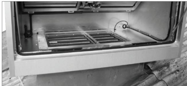
Fig. 29: Ugrađen odsisni filter
